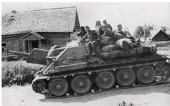
The T-34/85II was introduced in 1947 with improvements to the transmission, armour arrangement, and better fire control and vision devices. Used extensively in the Korean War, it initially equipped the Warsaw Pact nations and was exported throughout the world.
